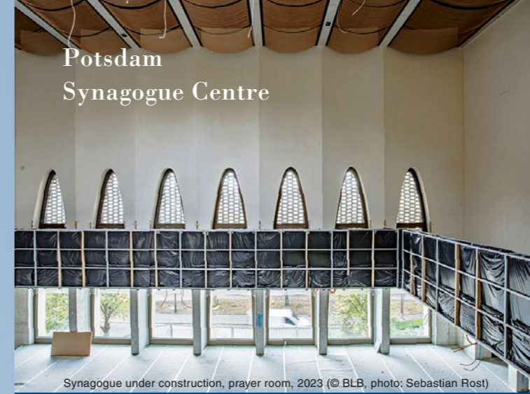
Synagogue under construction, prayer room, 2023 (© BLB, photo: Sebastian Rost)
