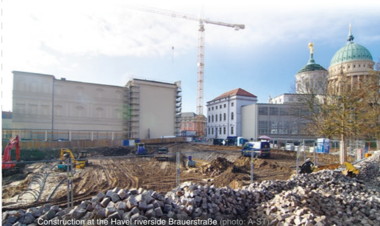
Construction at the Havel riverside Brauerstraße (photo: A-ST)
