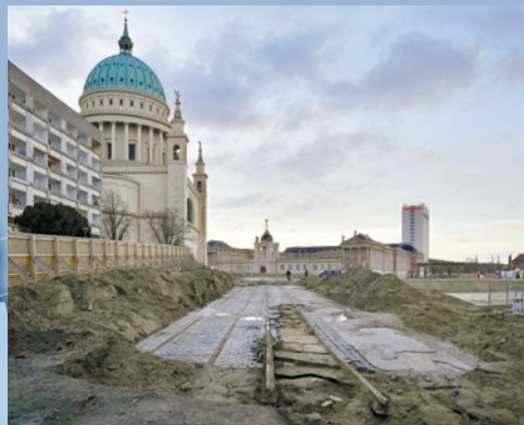
Historical pavement west of St. Nicholas Church
